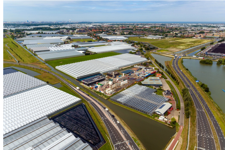
Geothermie ©Trias Westland
